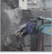
CUT Multi Crushers have concrete cracking wedges on the jaw ends and steel cutting blades in the center at the pivot of the jaws. They can be used for both concrete breaking and steel cutting applications.
