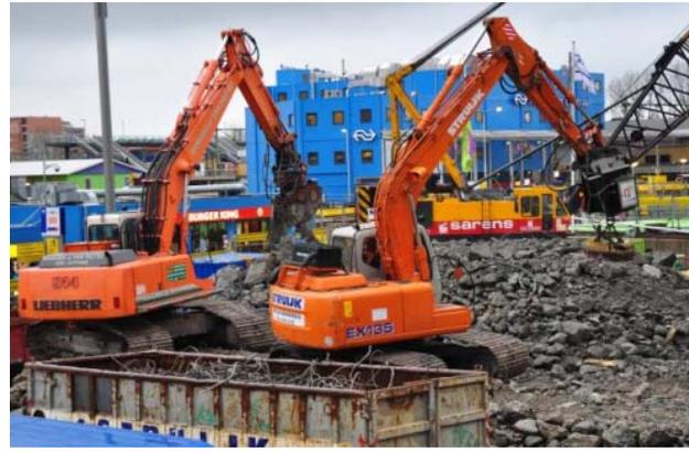
Excavators on the stockpile-this is where the demolition material is reduced to recyclable sizes and the reinforcement steel separated by magnet.
