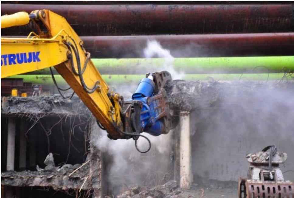
Demolition with a wide mouth and strong jaws – on the boom of the Komatsu PC 450 LC 8 crawler excavator are the free-rotating, 6.4 t OKADA TSW 1800 VFR concrete crushers – the crushers have a quick-entry valve for accelerated work speed.
