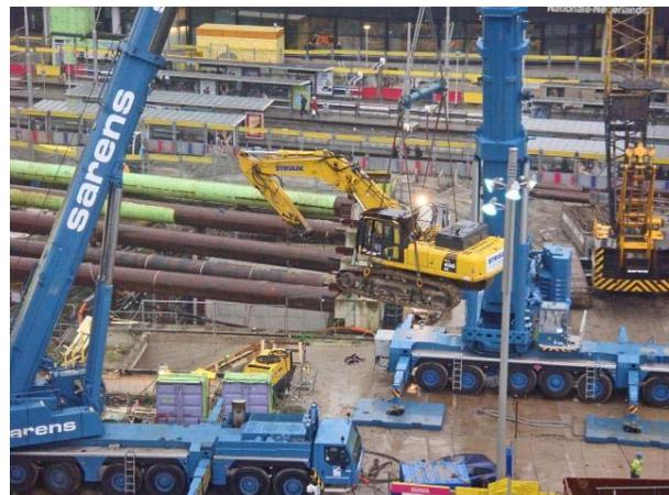
45t excavator on the extended booms of two Demag AC 500-2 and AC700 telescopicmobile cranes (photo from Struijk)
